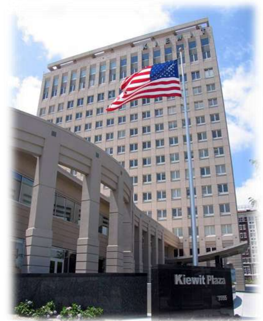
Kiewit Corporate Headquarters Omaha, NE
